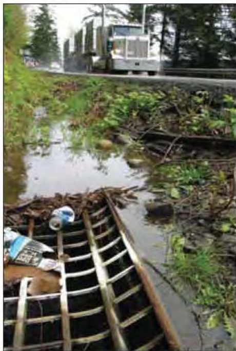
After a rain, stormwater runoff containing nutrients, bacteria, sediment and toxic chemicals collects in roadside ditches, runs into culverts, and flows into Hood Canal.
