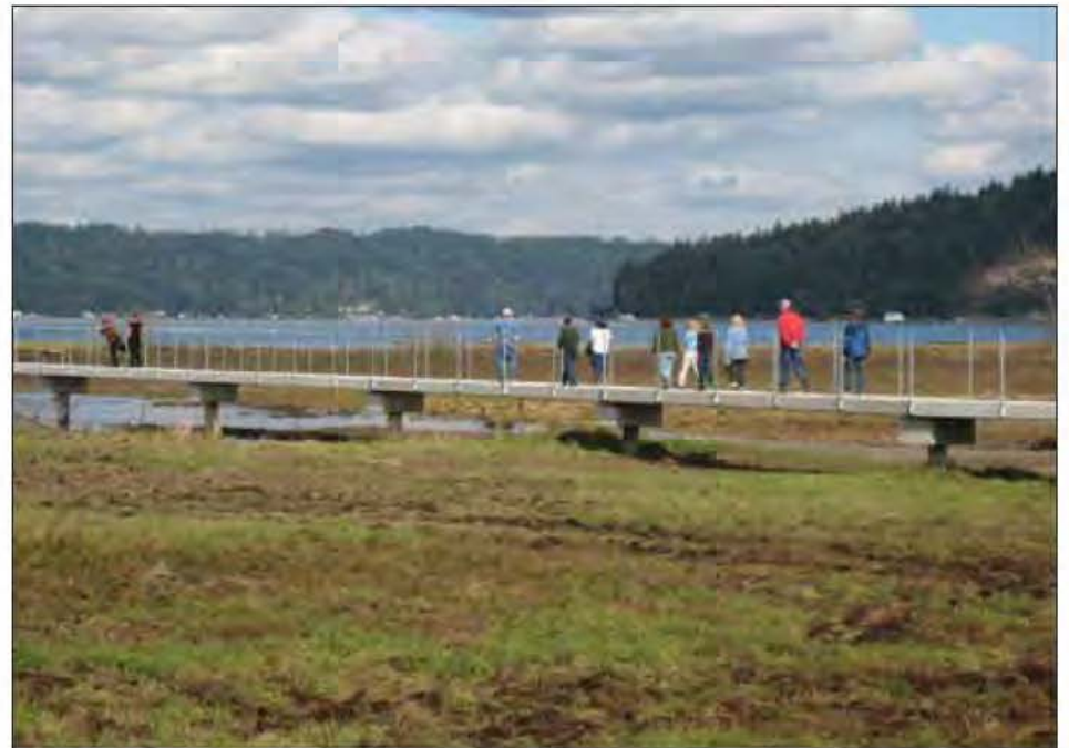
An elevated walkway allows people to appreciate first-hand the results of the Skokomish River Estuary restoration project.
