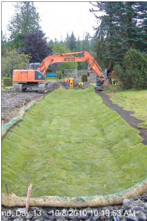
Stormwater improvements underway in Mason County.
